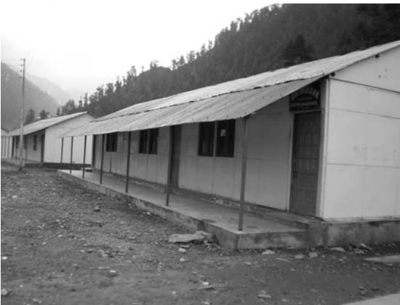
Meeting with the J&K administration, preparations for rehabilitation and completion of the school building
